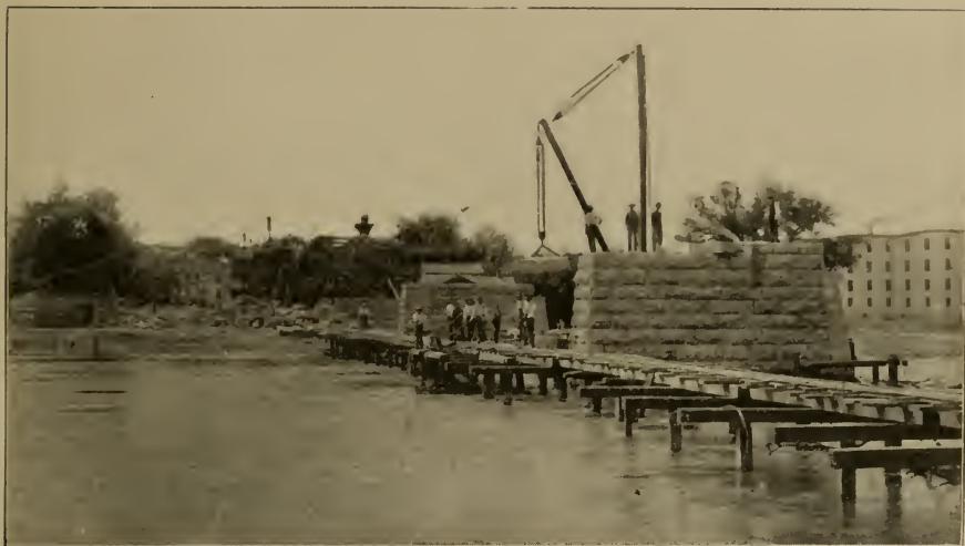
MORGAN STREET BRIDGE FOUNDATION—ROCKFORD, ILLINOIS.
